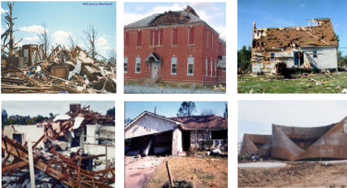
Figure 2 : Damage or Destruction of Structures
