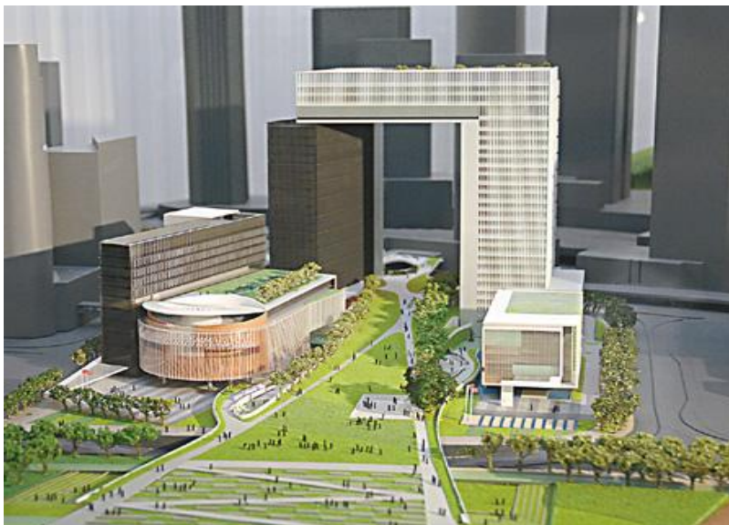
Figure 16. The Tamar design with the whole hole in it for better air ventilation.
