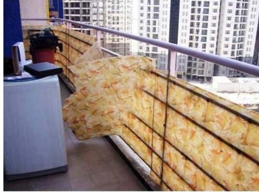
Photo.4 Wind damage to parapet of tall building
