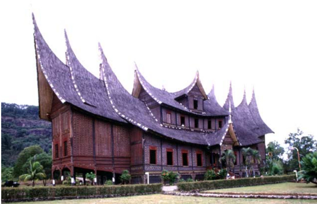
Figure 11. Traditional Minangkabau House (West Sumatera): seismic-proof but not wind-proof
